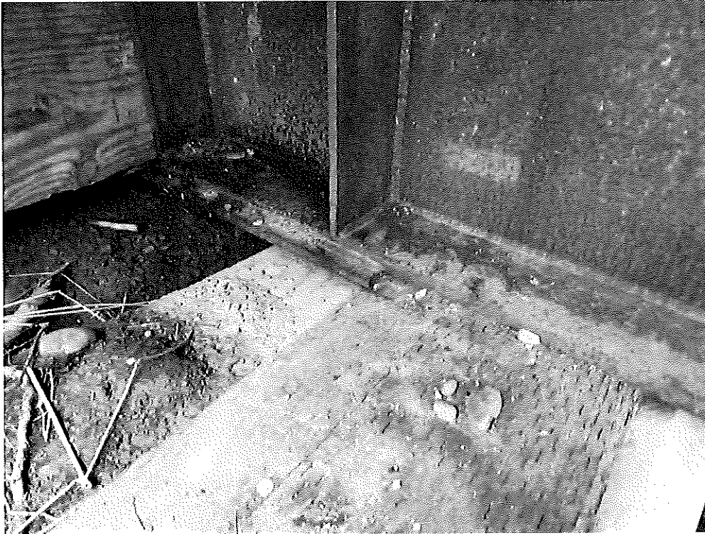
Figure 3: Lowchain upstream off-centre bearing
