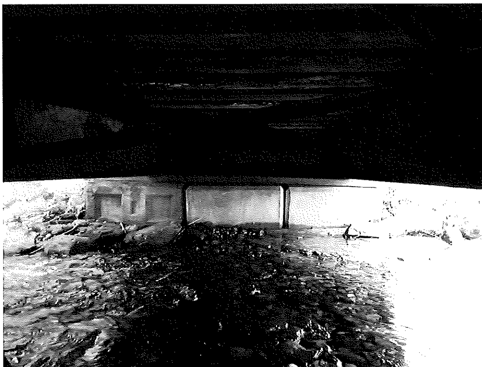
Figure 8: Intermediate Diaphragm Brace
