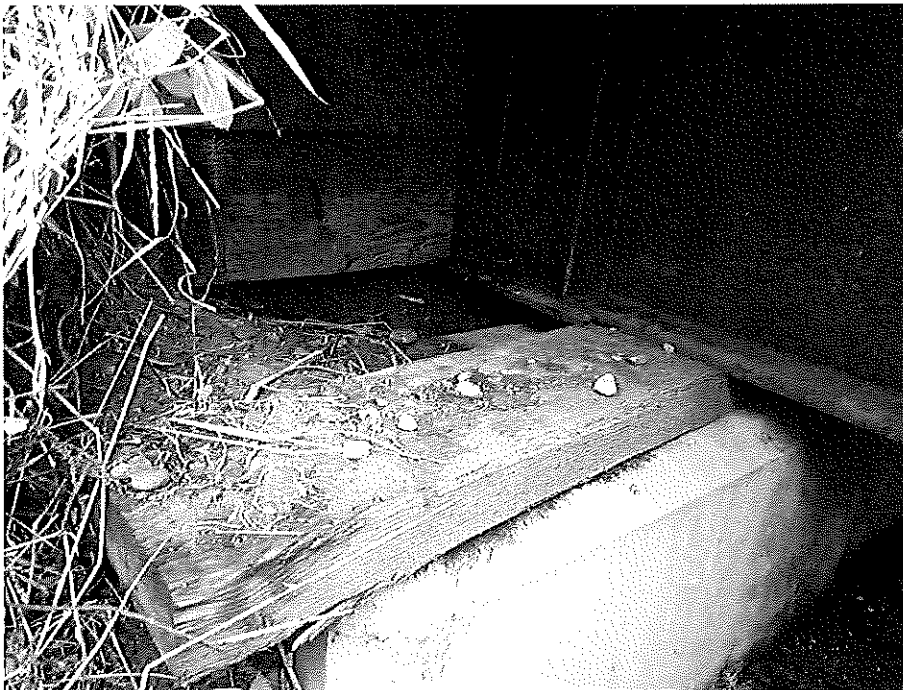
Figure 2: Lowchain upstream Skewed timber cap
