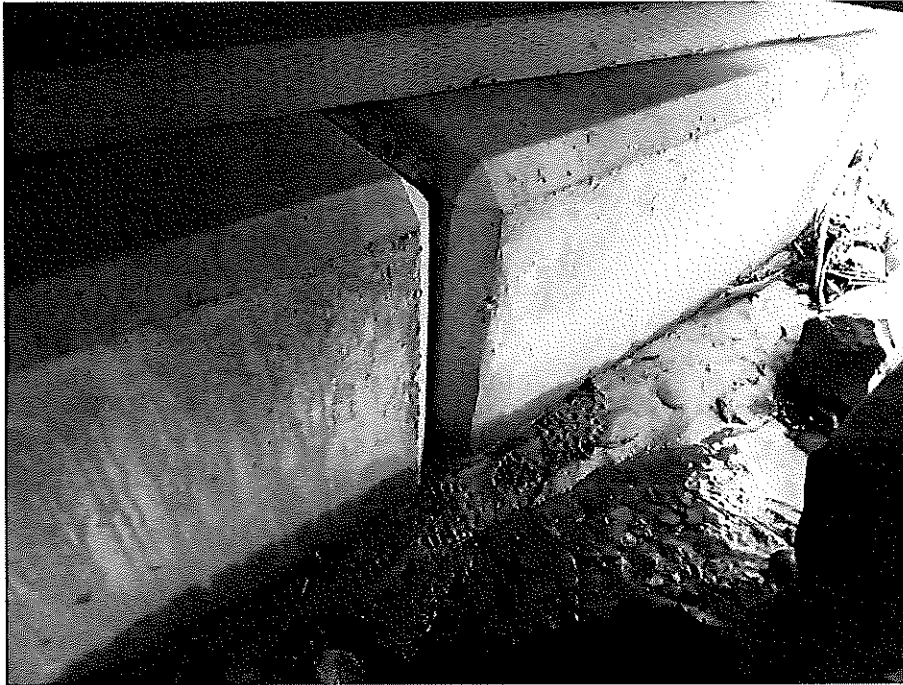
Figure: Highchain abutment shifting
